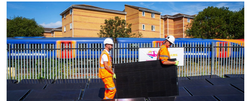
Installation of Solar Panels by Network Rail
